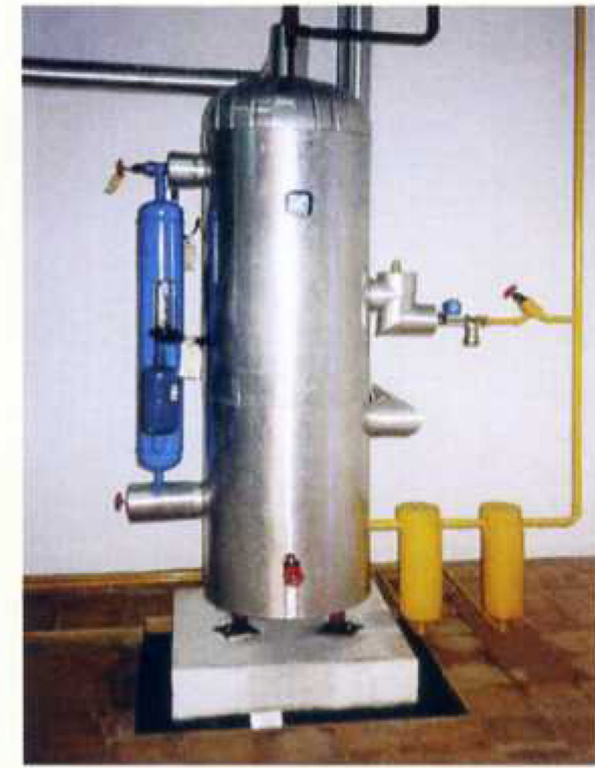
Vertical Intermediate Cooler Vessel
